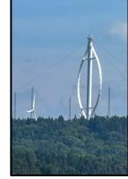
by far the largest VAWT constructed. The Éole turbine had a direct synchronous generator based in the ground. The total cost of turbine was 27.5 million dollar which was huge investment at
